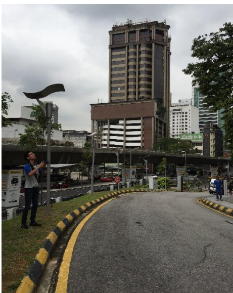
Entry from Jalan Tun Perak (1)
