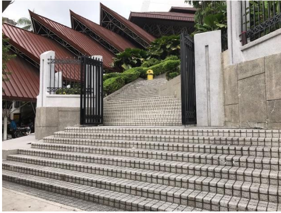
The entrance stairs connecting to the lobby area
