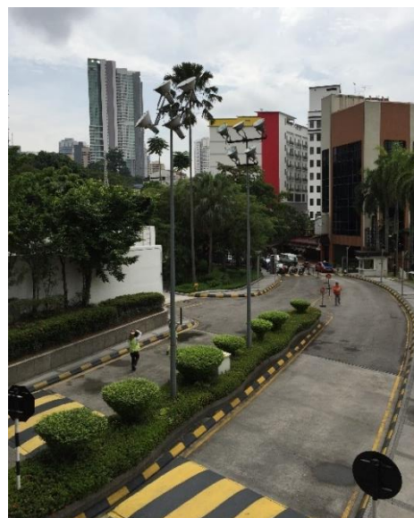
Entry from Jalan Pudu Lama (2)
